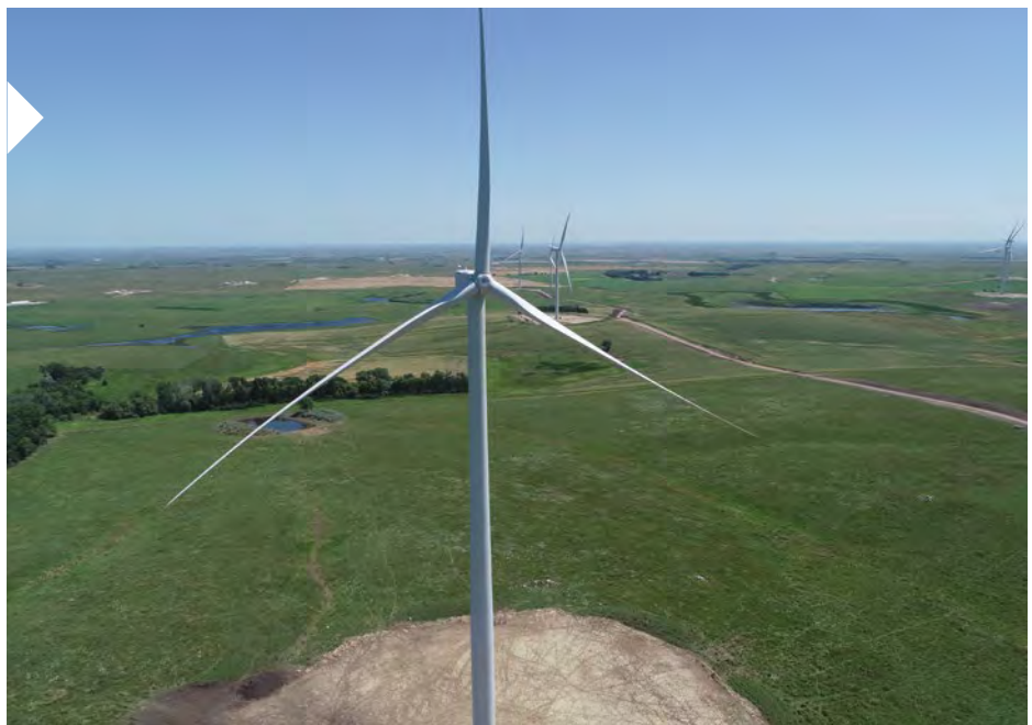
Crocker Wind Farm, National Grid Renewables, South Dakota, US
