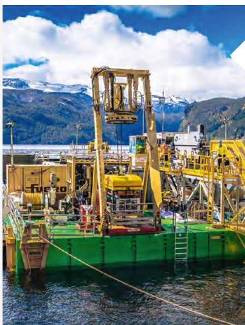
North Sea Link – specialist barge laying undersea cable in Norway
