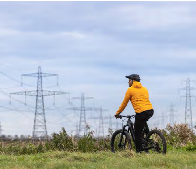
The Nemo Link Interconnector that runs between Britain and Belgium powers the Richborough and Canterbury, high-voltage overhead line.
