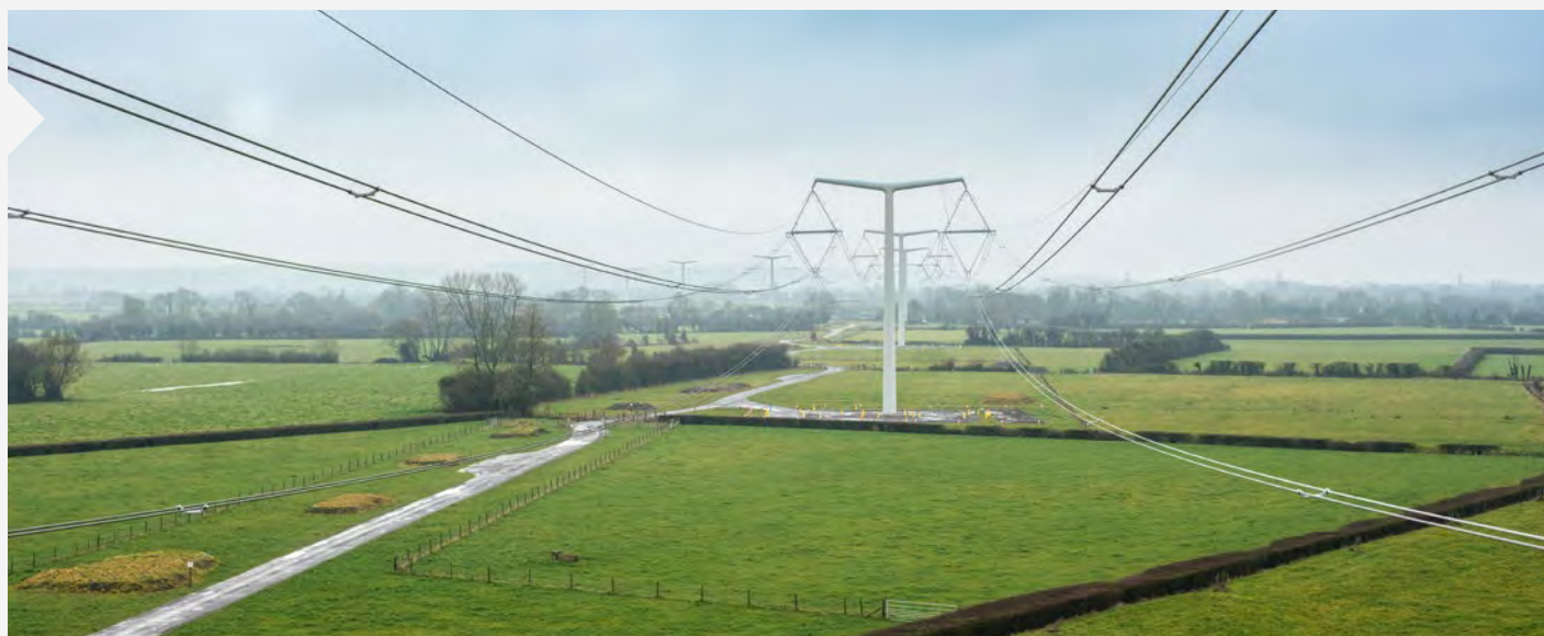
The world's first row of T-pylons, Hinckley Connection Project, UK
